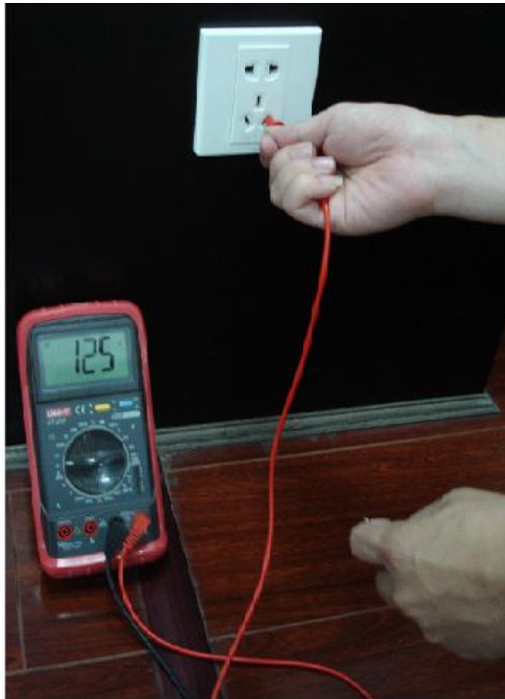
Appendix Figure 7-6 Check live cable connection
